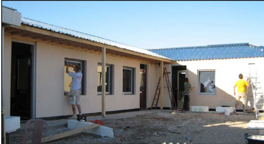
NEW ECD CENTRE FOR ZAMUKHANYO COMPLETED IN APRIL 2007
